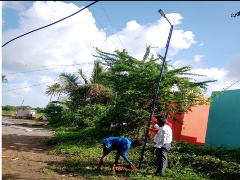
B) Installation of LED street lamp on metallic post
